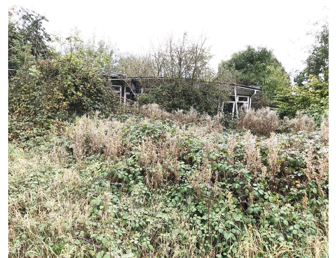
The site is overgrown with weeds and shrubs
