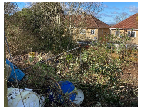
Rear view of the site with the overgrown bank and waste detritus visible
