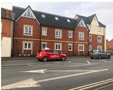
Existing Carnival Court apartments building viewed from Taunton Road.
