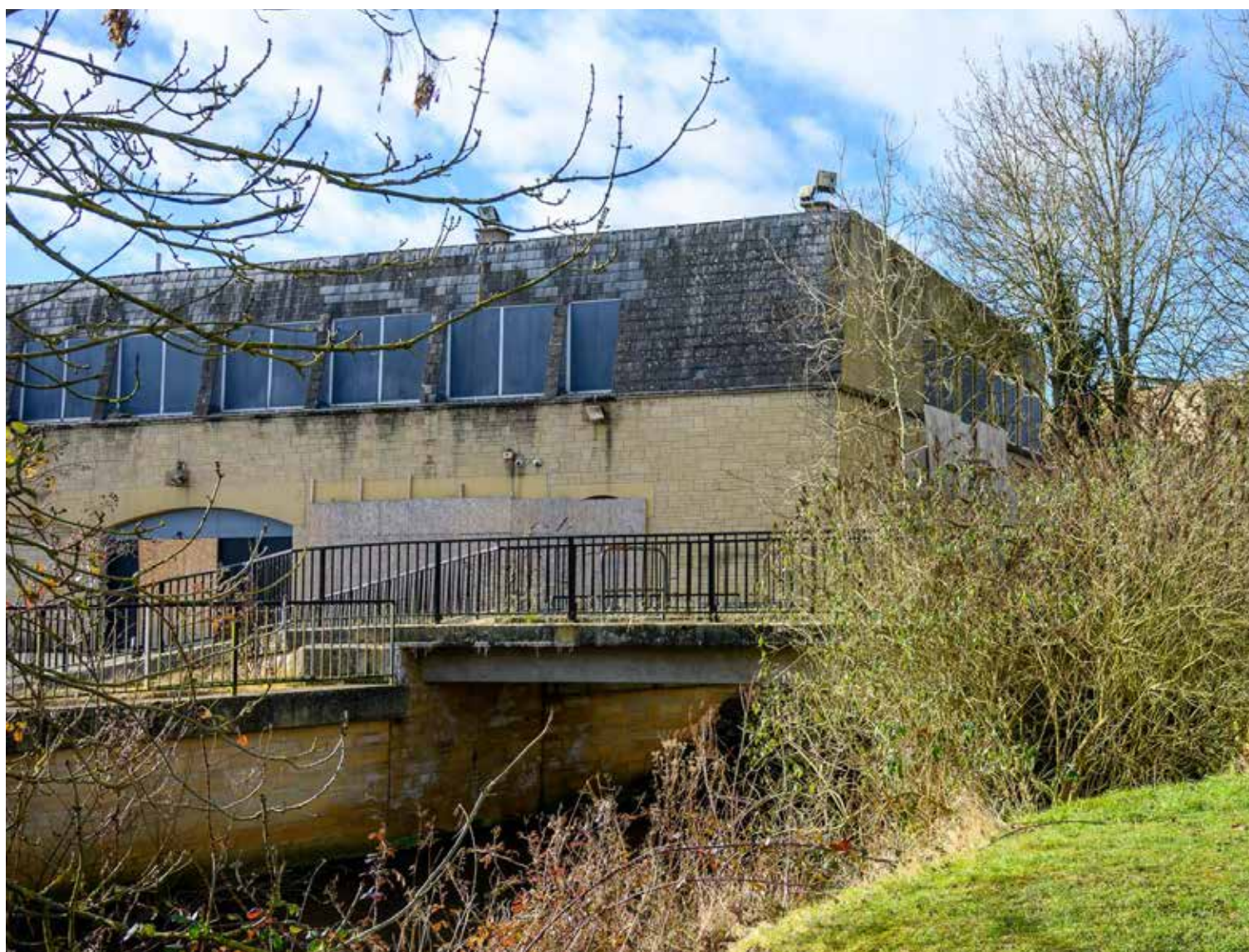
Pedestrian Bridge / River Marden connecting the northern and southern parts of the site
