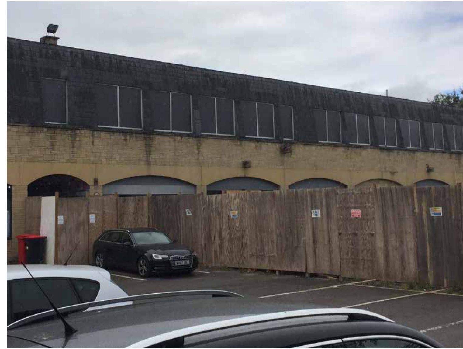
View of Car Park on Co-op building – southern part of the site
