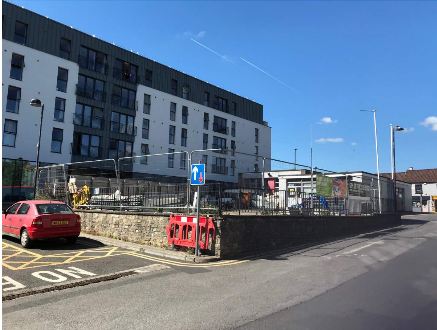
Figure 1.1: View of the site from east (looking from the entrance to Civic Centre Car Park). Existing stone retaining wall to the eastern boundary of the site - site is 1.35m higher than the unadopted private road ground level.
