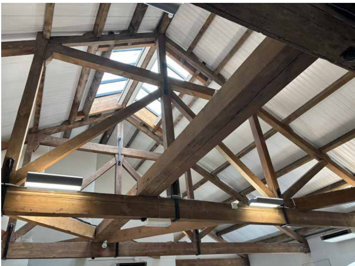
Photographs of existing trusses. Green dashed line indicates areas where diagonal bracing is removed to accommodate new second floor living space
