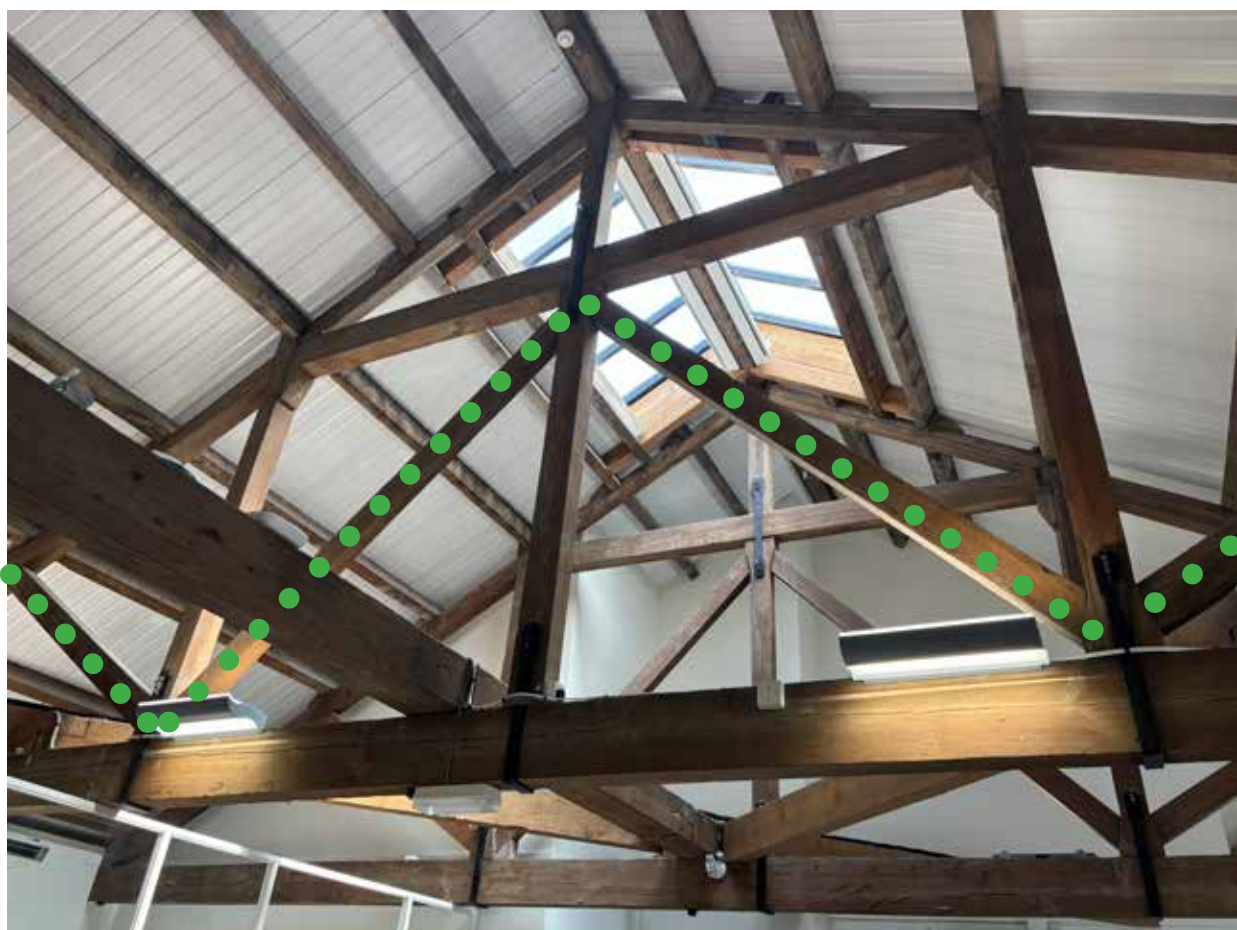
Photographs of existing trusses. Green dashed line indicates areas where diagonal bracing is removed to accommodate new second floor living space
